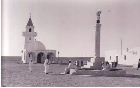
Figure 13a. Mosque built during the Italian Period (Buhlfaia, 2006)
