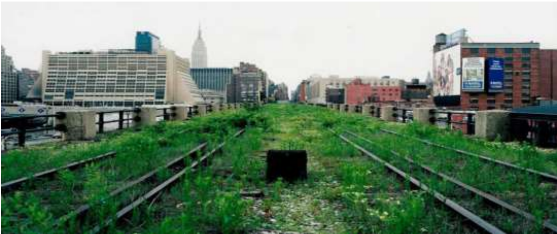
Figure 4: The High-Line before restoration (thehighline.org)
