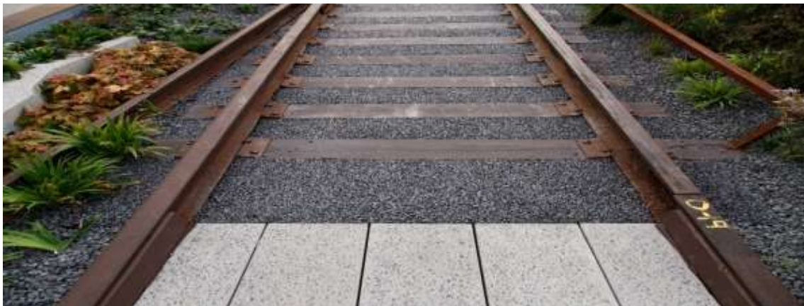
Figure 9: Original rails lined with loose stone gravel bonded with aggregate, smooth enough for the physically disabled to use (thehighline.org)
