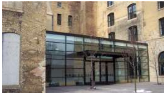
Figure 31: Historical masonry facade in Leipzig, Germany
