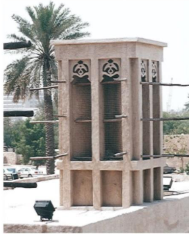
Figure 2: Al- Barajeel as appear at the roof of the buildings (Alkhalidi, 2013).
