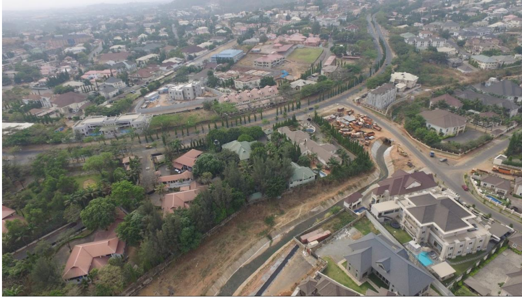
Figure 10. Maitama District, Resource: (Google Earth, 2024)
