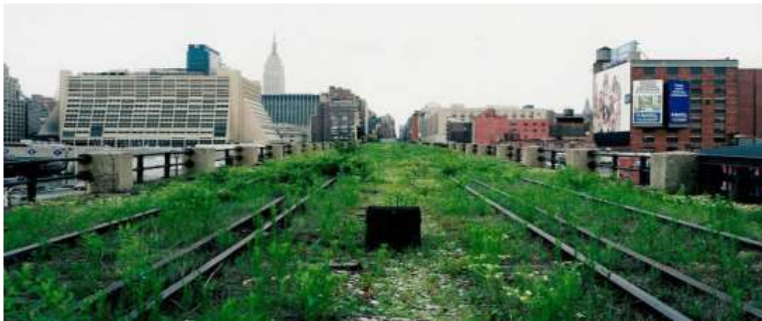
Figure 4: The High-Line before restoration (thehighline.org)
