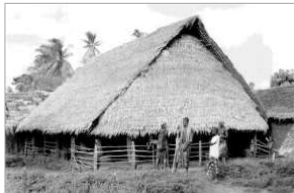
Figure 3: A steep roof (Ikebude, 2009)
