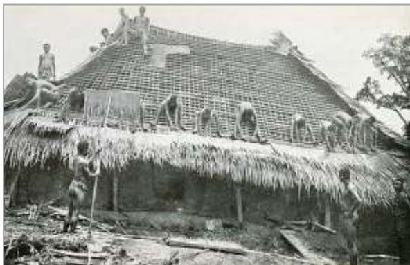
Figure 2: Roof construction (google.com)
