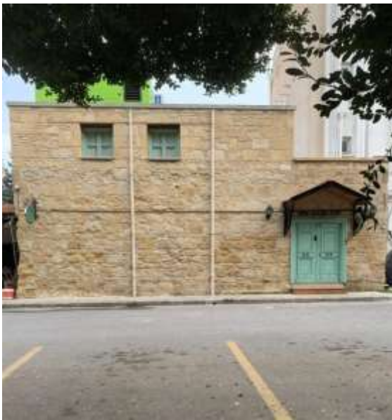
Figure 3. Ottoman period stone house with no windows on the ground floor for privacy (Author N.U)
