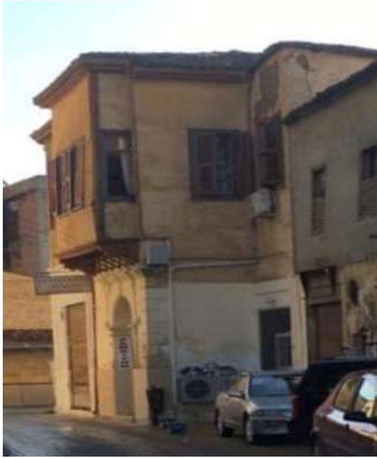
Figure 1. Stone on the ground floor wall adobe on the first floor walls of Ottoman house with bay window (Author, N.U)
