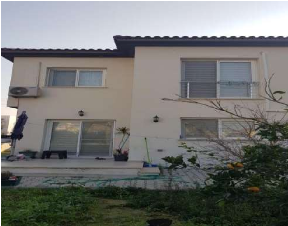
Figure 21: Back facade facing West (Author, N.U)
