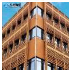
Figure 7: Building Design Decorative Terracotta Baguette Louver
