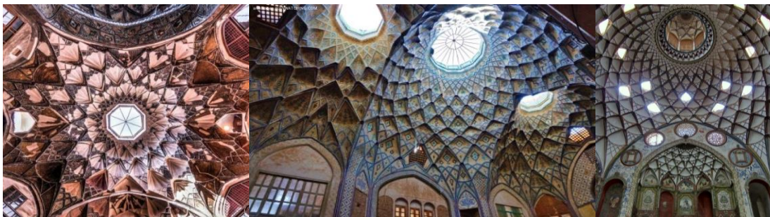
Figure 9: Karbandi and Muqrans on the dome of the buildings, (Saljoughinejad & Sharifabad, 2015).
