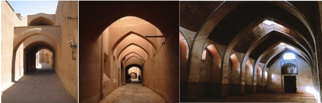
Figure 4: Saradaq & Sabat, the shading element of the narrow street in tropical climate cities, (Akbarzadeh, 2016)
