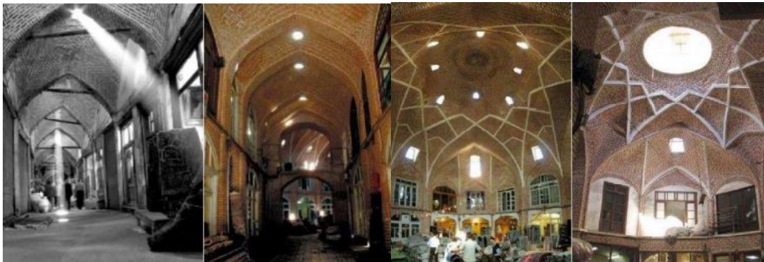
Figure 15: Dome in traditional bazaars in Islamic cities like Iran are seen from the exterior and arch pathways from the inside (Shalchi, 2013)
