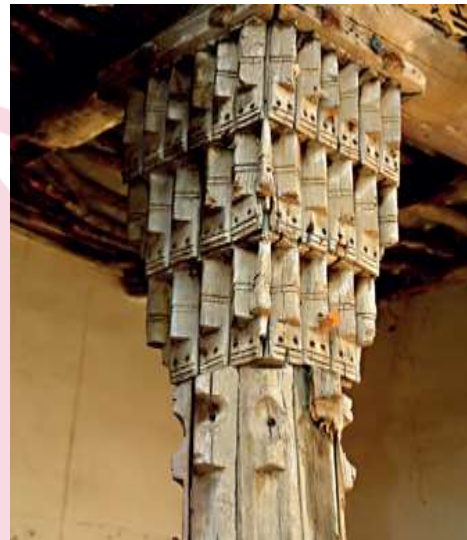
Figure 10. Timber columns of porticoes in Citadel (HCECR, 2012b).
