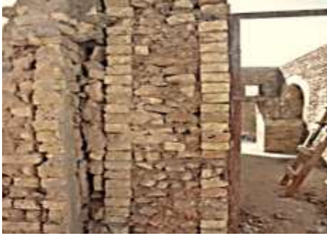
Figure 11. Section of wall in Citadel (HCECR, 2012b).
