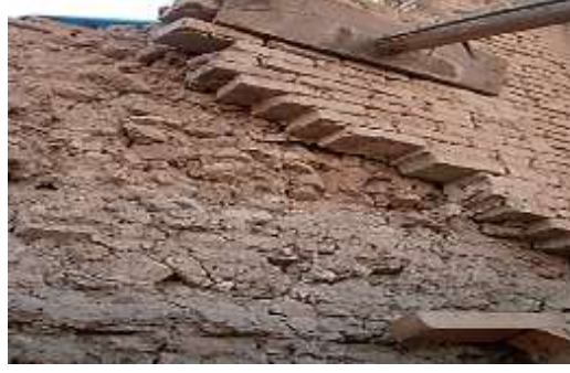
Figure 12. Wall construction in Citadel (Palumbo, 2011).
