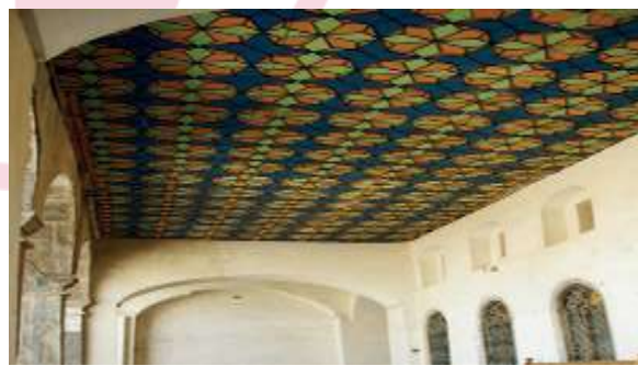
Figure 14. Dwelling roof of citadel restored in 1980 (Mirani, 2010).
