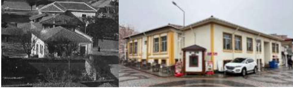
Figure 13a. South and east facade of the original building (Öztabak, 2015)
