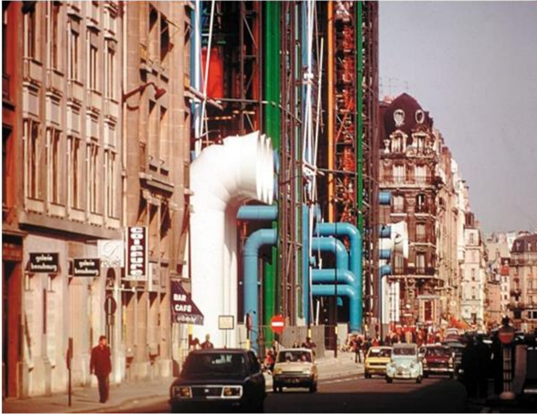
Figure 9: Color coded infrastructure and neighboring buildings ( https://www.dezeen.com/2017/01/31/renzo-piano-richard-rogers-photography-centre-pompidou-paris-40th-anniversary/ )
