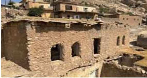
Figure 23. Used materials for construction in Old Akre (Ismael & Hasan, 2023).
