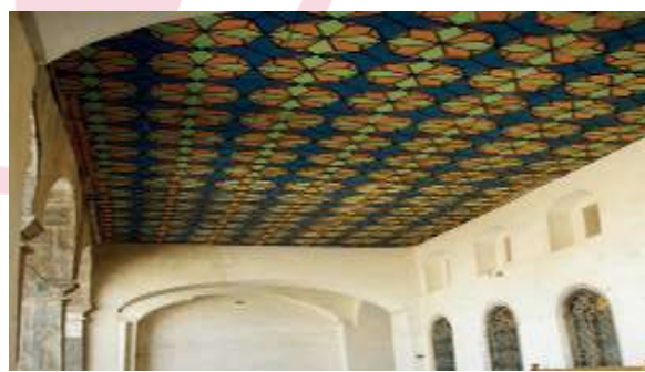
Figure 14. Dwelling roof of citadel restored in 1980 (Mirani, 2010).
