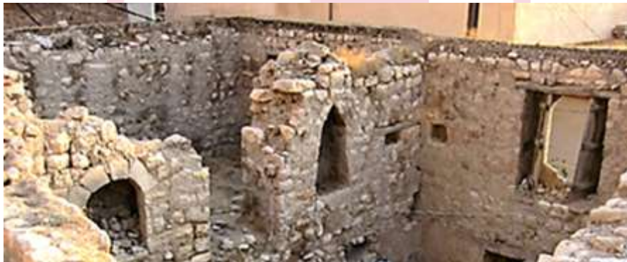
Figure 25. Wall construction of Akre (Spät, 2019).
