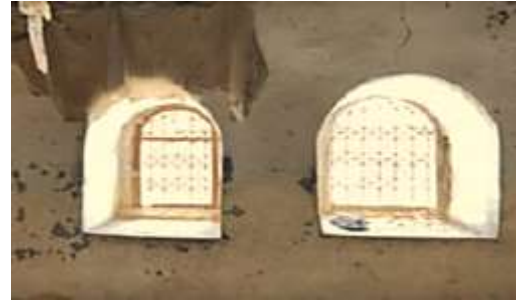
Figure 24. Lime plaster for interior finishes in Old Akre (Ismael & Hasan, 2023).
