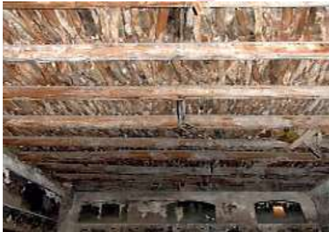
Figure 13. Dwelling roof of Citadel (HCECR, 2011).
