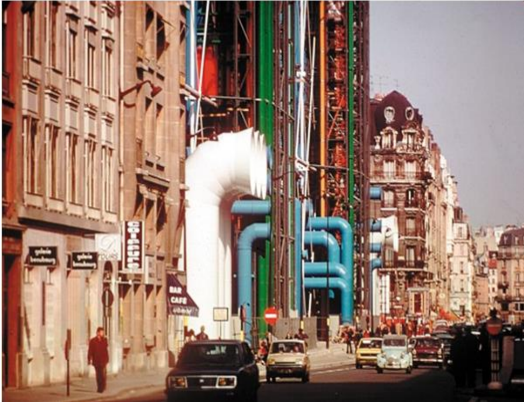
Figure 9: Color coded infrastructure and neighboring buildings ( https://www.dezeen.com/2017/01/31/renzo-piano-richard-rogers-photography-centre-pompidou-paris-40th-anniversary/ )
